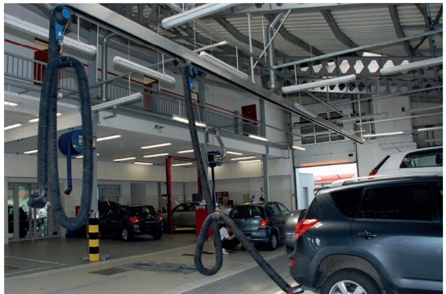
Technorail with 11000 Series Balancer Drop
